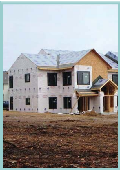
New Housing Development (Source: Hidden Valley Website)
